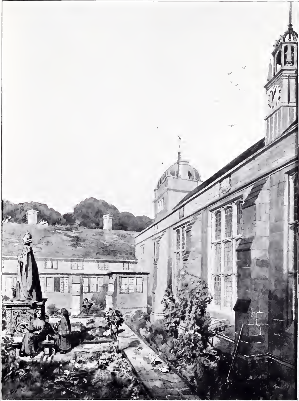
1393. Quadrangle, Queen Elizabeth Grammar School, Hexham, OLIVER LEESON AND WOOD, Architects. (For Plan, see p. 15.)
